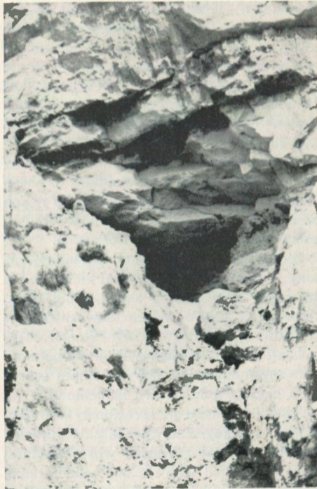
Figure 5. The downstream end of the Tunnel at Mason Draw.
